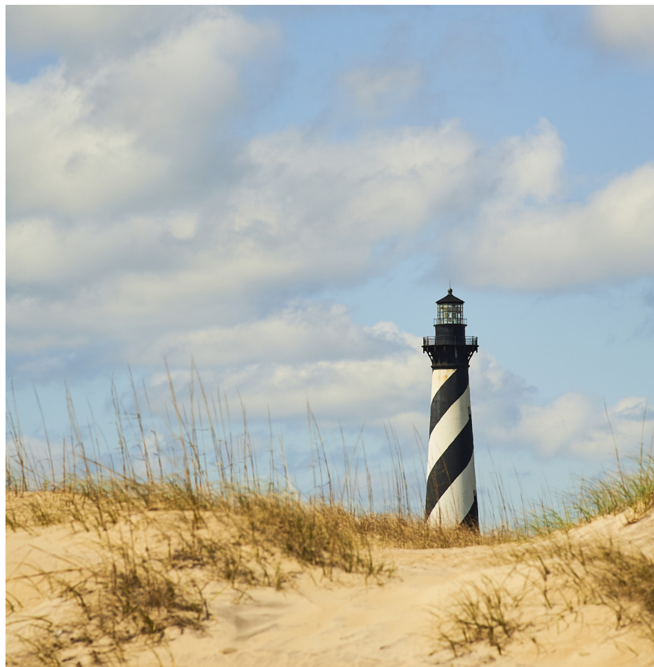
Follow the restoration of the iconic Cape Hatteras Lighthouse at: go.nps.gov/cahalighouserestoration
